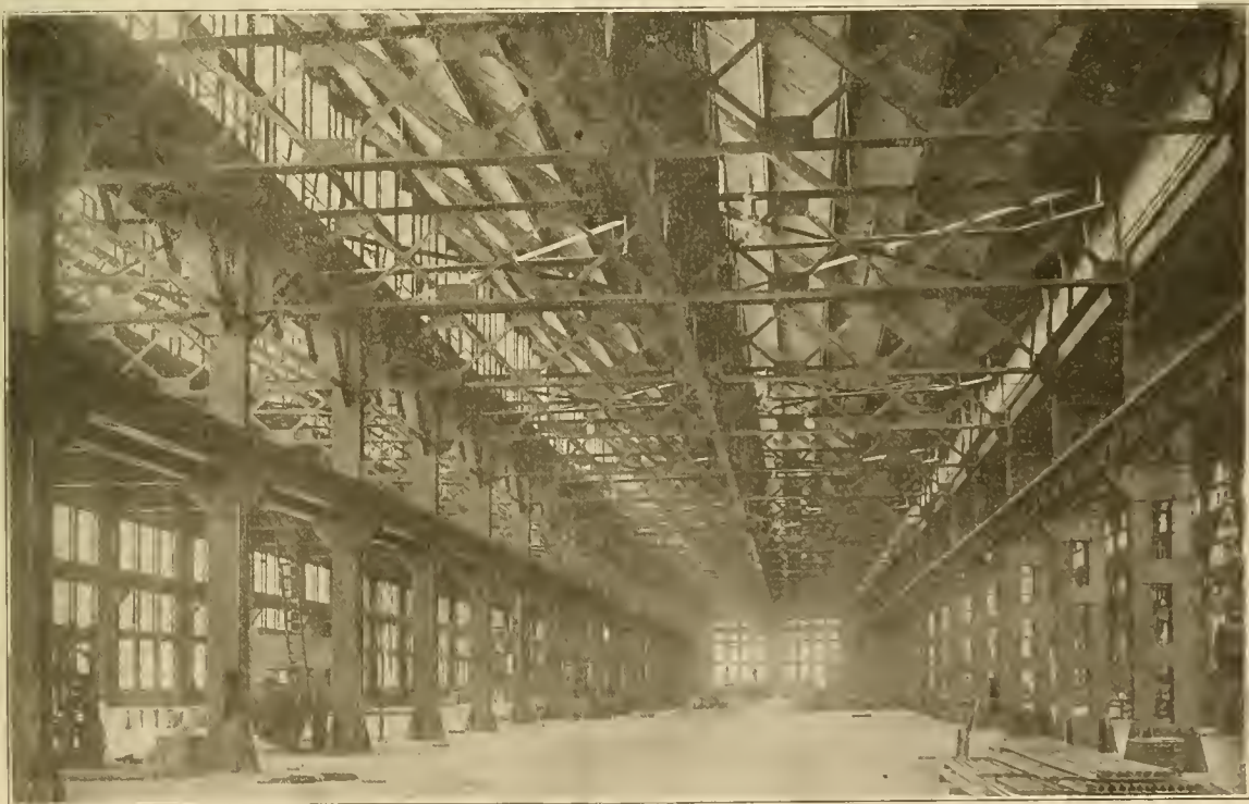
INTERIOR VIEW OF THE MACHINE SHOP, SHOWING DAYLIGHT LIGHTING EFFECT FROM THE SAW-TOOTH WINDOWS. MCKEES ROCKS SHOPS.—PITTSBURGH & LAKE ERIE RAILROAD.
